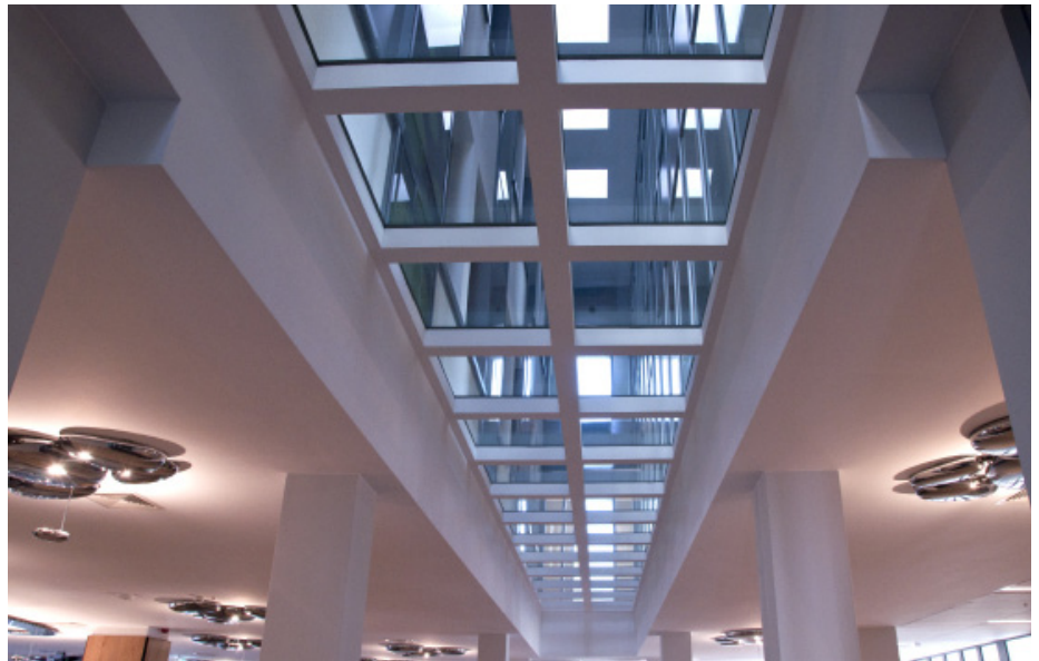
▲ Clinical Hospital of the Military Medical Institute in Warsaw. POLFLAM ® F REI 60 was used for the internal ceilings, light-saturating the main hall.
