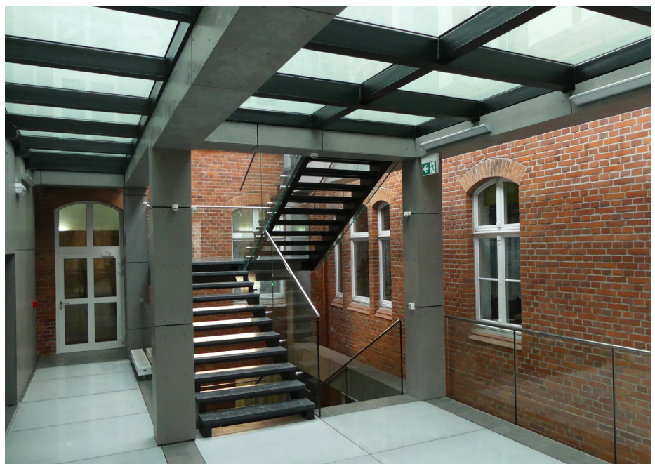
▼ Oskar Kolberg Music School in Szczecinek. The staircase ceilings of two floors have POLFLAM ® F REI 60 glass.
