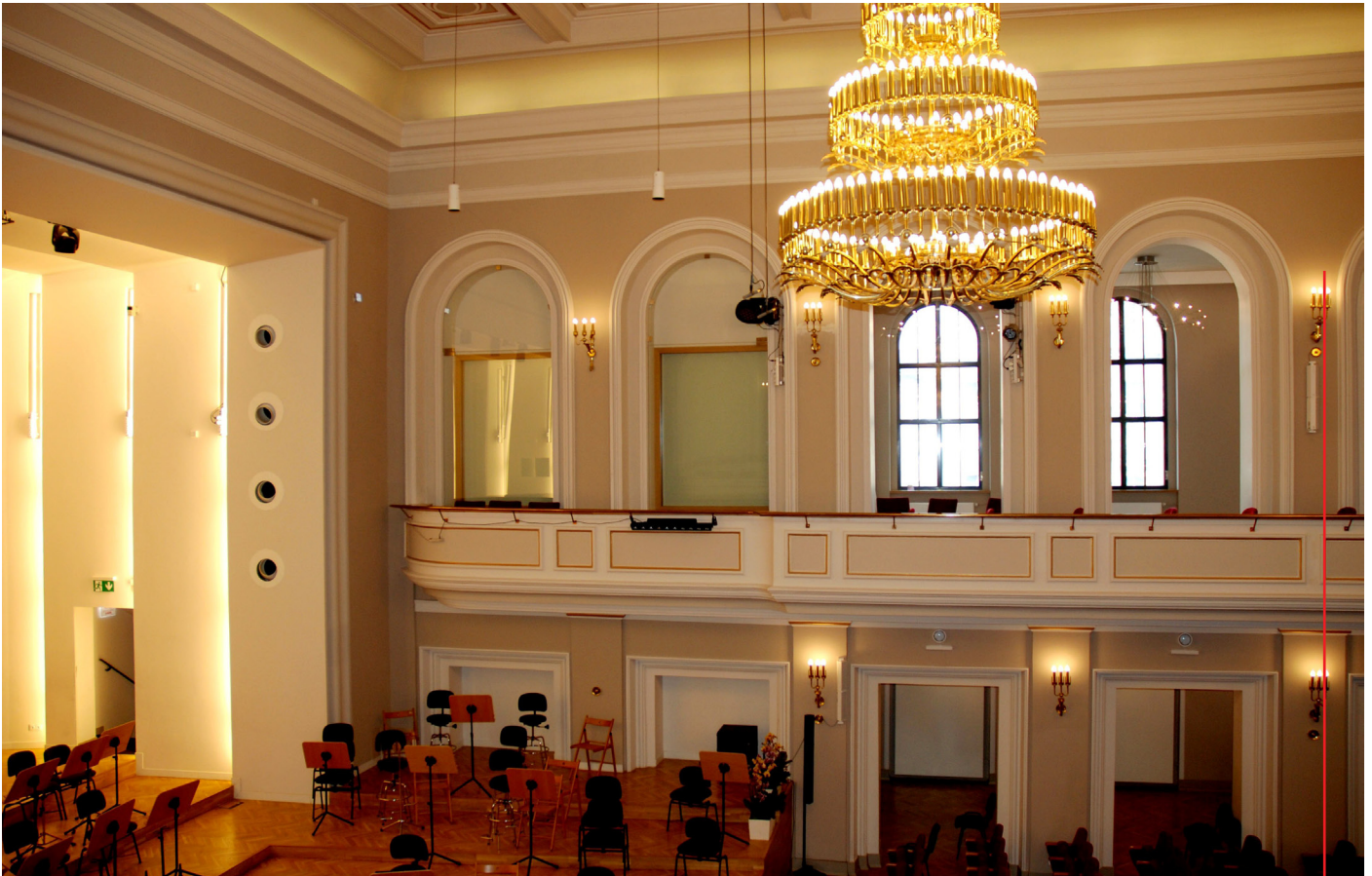
Polflam's fire-resistant glass placed in the arcades protects the Silesian Philharmonic's Recording Studio located right behind the wall by providing an adequate level of sound proofing..
