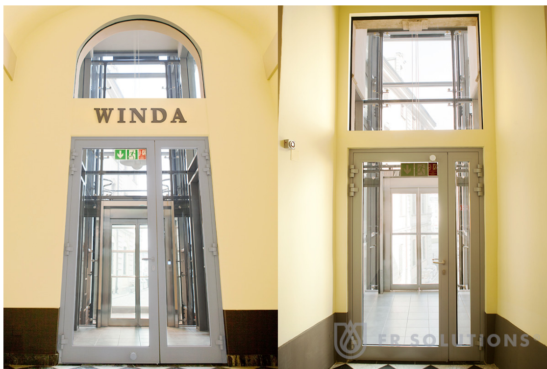
FR system of fire-resistance class EI 120 was used in the building of the University of Wrocław. Thanks to the application, the narrow corridor now gets more light.
