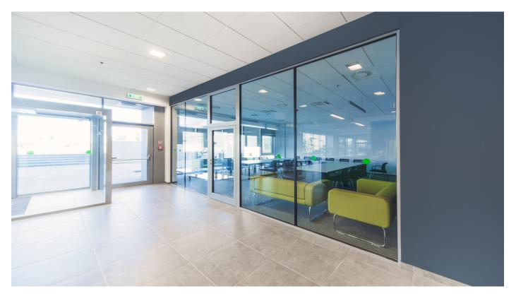
BR system allows for effective combining of clear and opaque glass pane in one fire protection partition as well as fire protection classless doors
