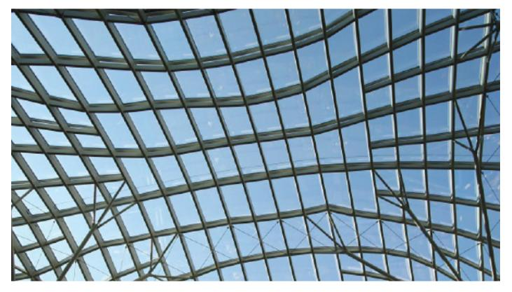
The POLFLAM<sup>®</sup> glass panels inside the frames can be as large as 2654 x 1174 mm.
