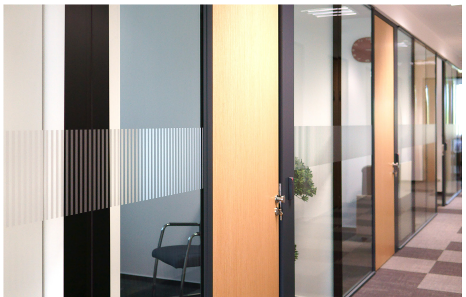
Using digital printing ceramic paint can be applied on glass to allow obtaining text or drawings, including 3D-effect images.
