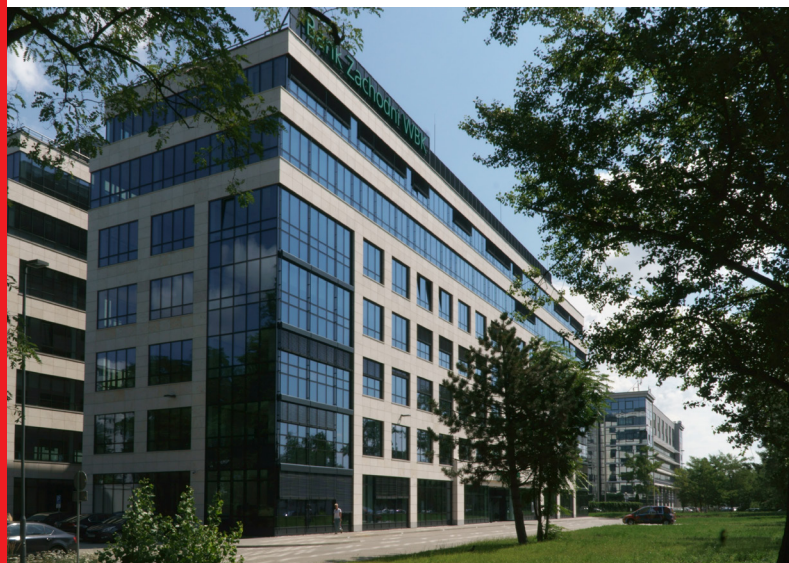
Bank Zachodni WBK – head office in Wrocław. POLFLAM glass was used in the facade of the building with the required fire resistance
