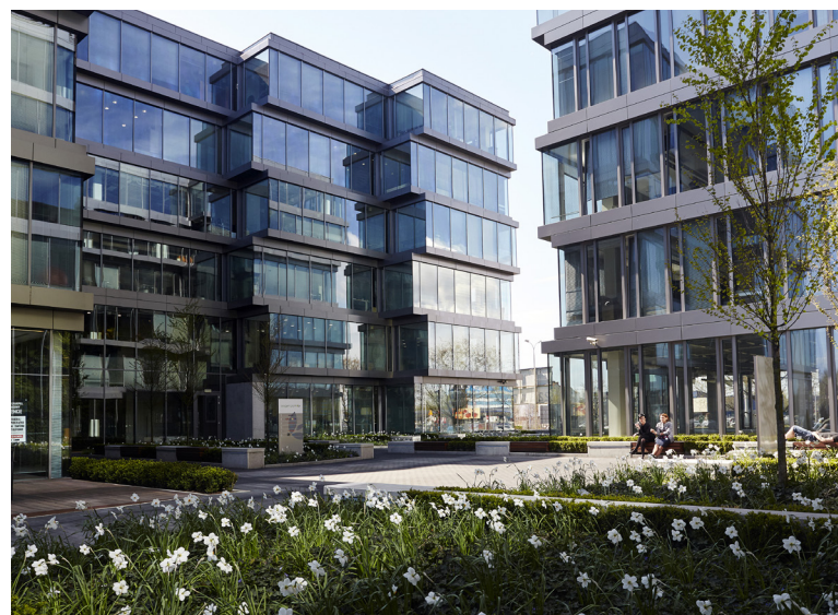
POLFLAM glass in the facade of Oxygen Park: a modern office complex in the business area of Warsaw
