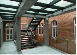
Glass ceilings with fire resistance make it possible to saturate with natural light the interiors as difficult as staircases, internal courtyards or rooms below the ground level. In the photo:
