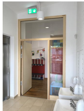
▲ POLFLAM ® fire-resistant glass in the door and wooden windows with natural finishing at the school premises in Kayl, Luxembourg
