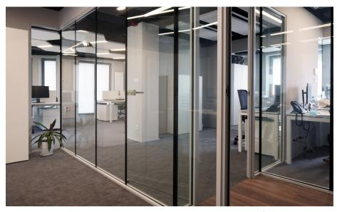
Our frameless glazing system allows creating interior glazing systems without visible vertical profiles separating the panes.
