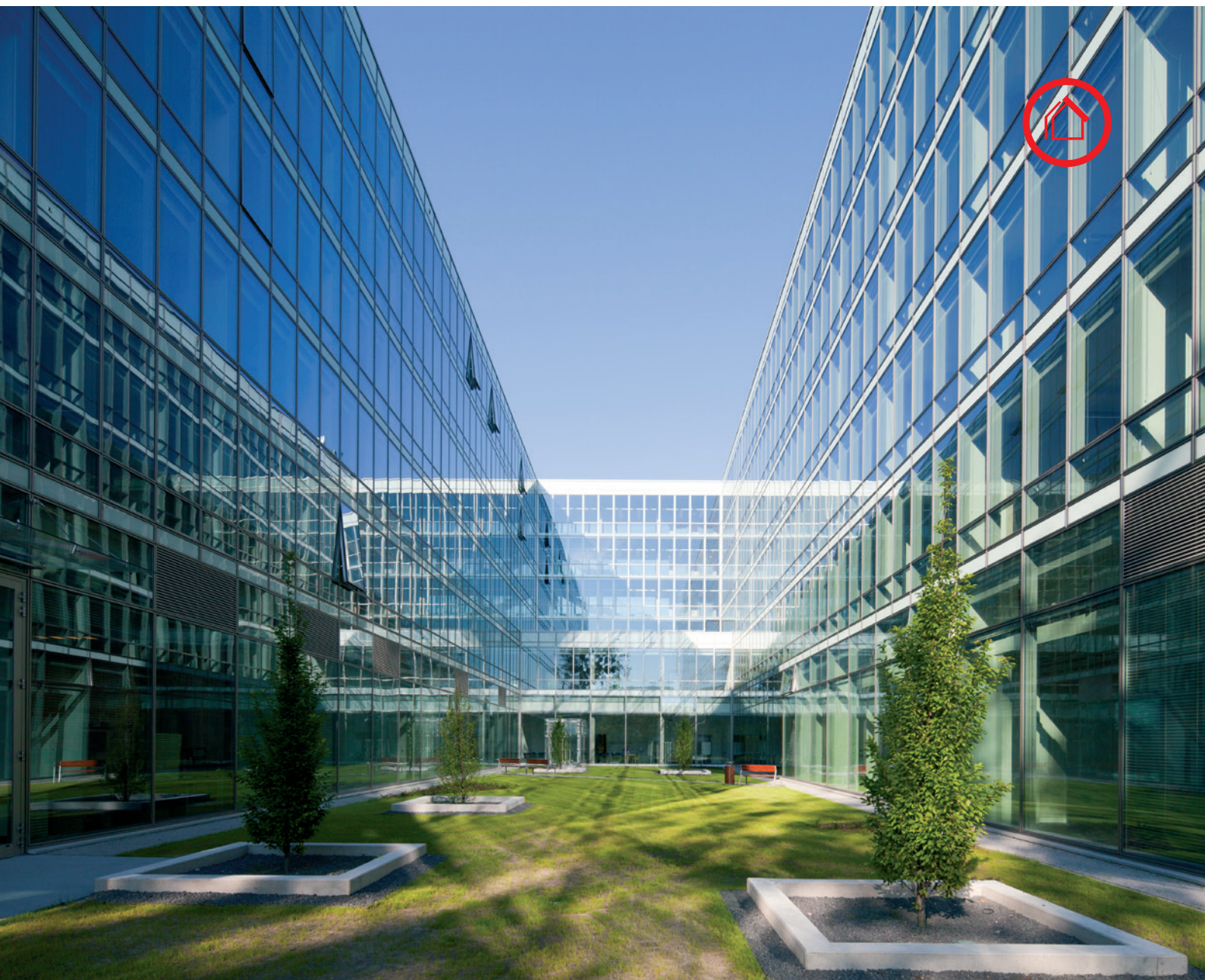
Curtainwall, class EI 60 at the Pomorski Science and Technology Park in Gdynia
