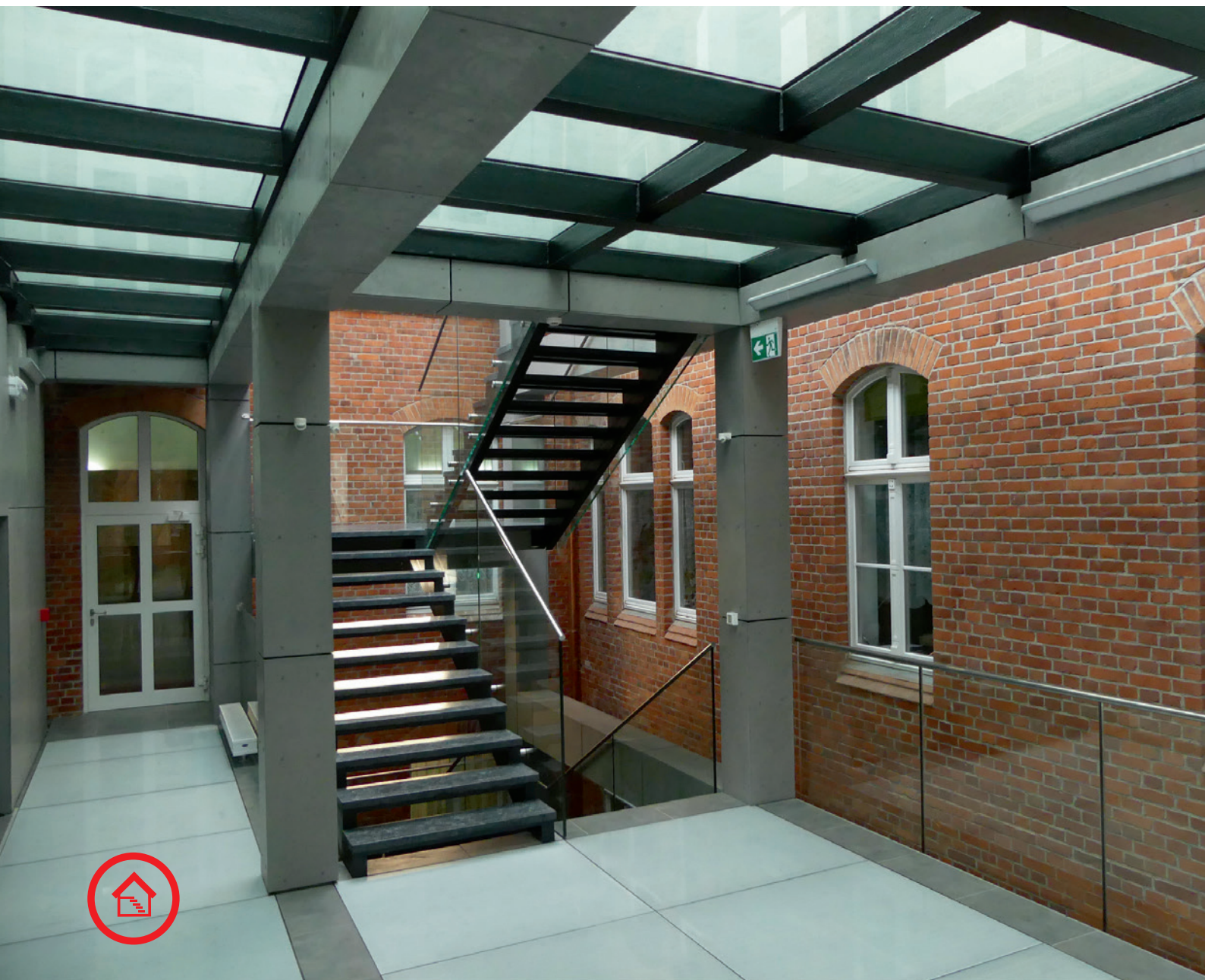
Ceilings with POLFLAM F glass of the REI 60 class applied in the two landings of the staircase at Oskar Kolberg Music School in Szczecinek.
